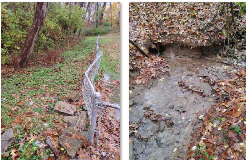
Figure 7 – Grass swale behind 714 Vincent Drive
