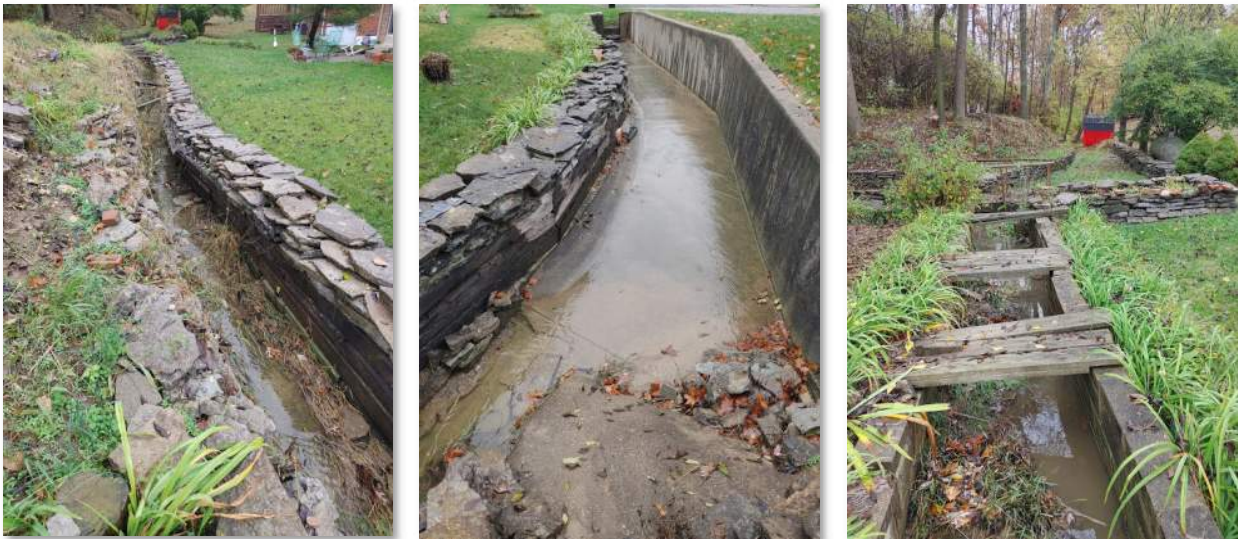
Figure 6 – Paved, rock-lined channel behind 716 and 718 Vincent Dr
