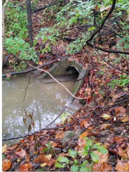
Figure 3 – Headwall at 748 Vincent Drive
