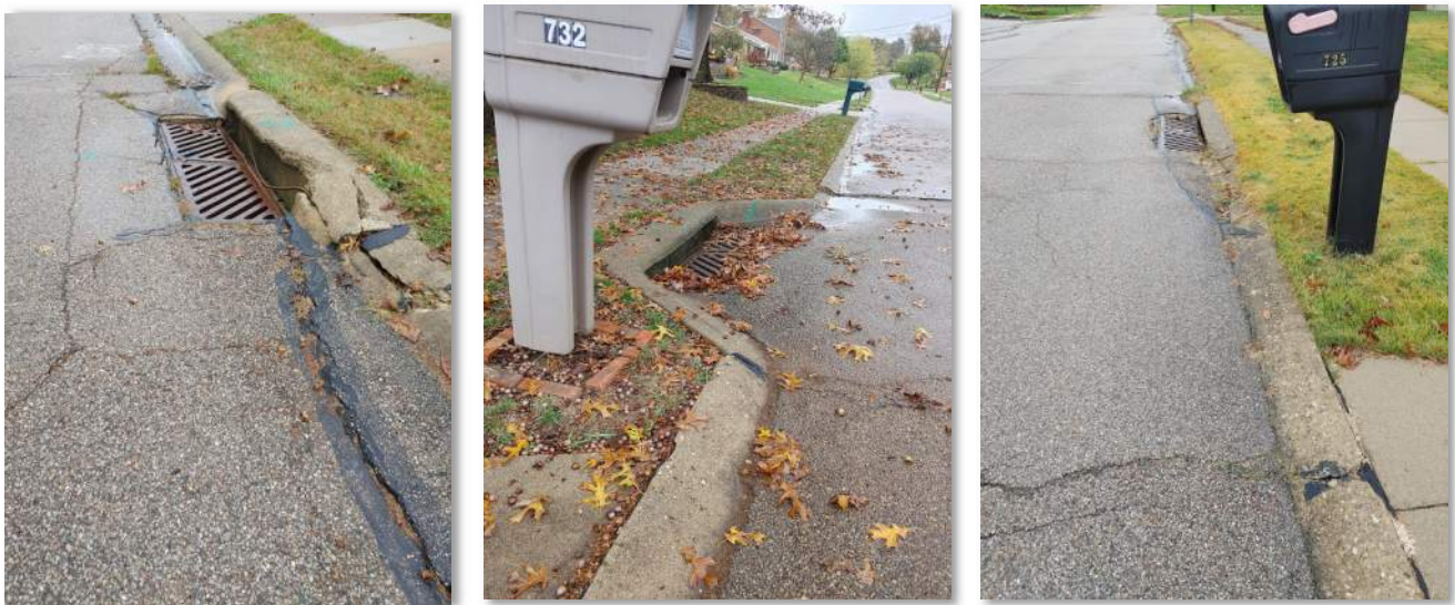
Figure 5 – Curb inlets along Vincent Drive
