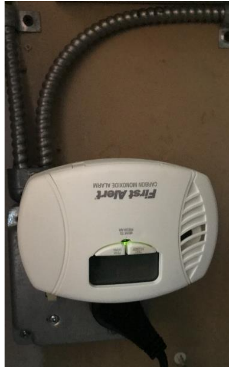
Figure FA2 - CO alarm unit
