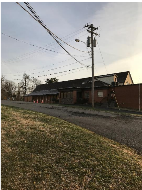
Figure EP3 - Electric utility service
