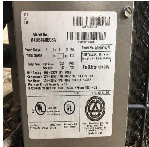
Figure 5 - Split-System AC Condensing Unit Tag (R-22)
